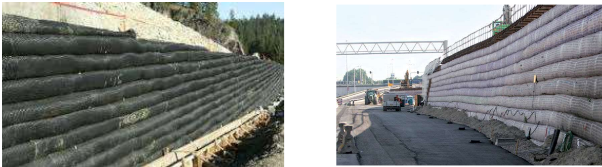
Figure 1: Typical wrapped face MSE walls
